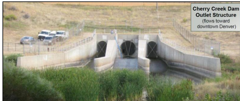
Figure 2: Cherry Creek Dam principal outlet (courtesy USACE)
